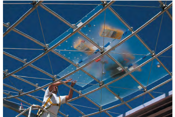
Figure 8: Placement of the glass panels (Photo: The Schubert Club)
