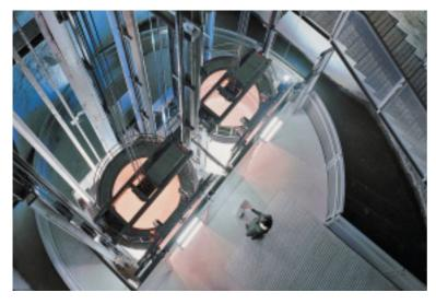
The lift frame is an open steel construction that is encased in glass at the exit levels.
