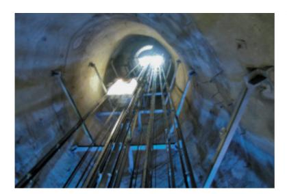
The two stainless steel lift cabins are clad on the outside with opaque acrylic sheet. Fitted between the stainless steel interior panelling and the acrylic sheet are fluorescent tubes that make the lifts look like lamps ascending and descending in the shaft. Stainless steel presents an interesting contrast to the rough hewn walls of the shaft and also stands up well to the damp atmosphere inside the hill.
