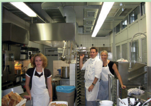
The kitchen of the institute's restaurant requires efficient air conditioning
